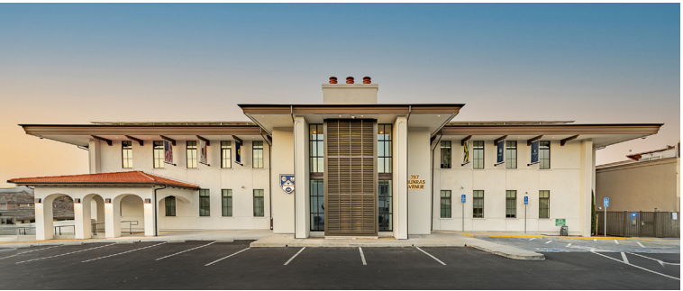
MIDDLEBURY INSTITUTE FOR INTERNATIONAL STUDIES STUDENT HOUSING Monterey, California Rehabilitating a 50-year-old building creates walkable student housing with a more contextually sensitive character.
