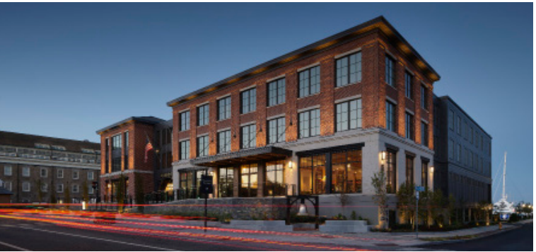
HAMMETTS WHARF Newport, RI Historic waterfront infill. Full design services from masterplanning, entitlement, design and construction.
